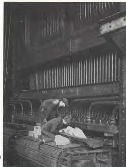
A Typical Chain-Grate stoker, under construction → (7)
